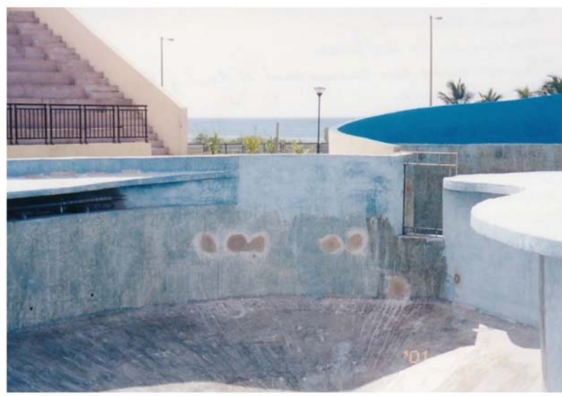
Waterproofing of pools in Dolphin show area in National Aquarium (Cuba)
