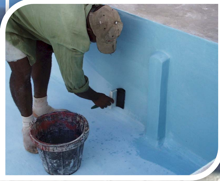
Waterproofing of "Espejo de Agua" funfair in National Aquarium (Cuba)
