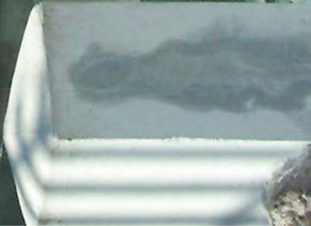
Waterproofing and protection of other areas and retaining water structures in National Aquarium (Cuba)
